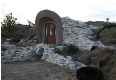
TRITON: 3 connected domes underground
