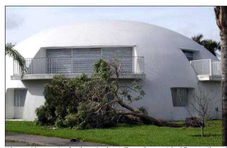
When not busy caring for the animals, staff members watched Frances through the domes' curved windows, made of a double layer of heavy plastic. "If we didn't have those windows, we would not have known that there was a hurricane out there," Valerie said. "That's how quiet it was inside. This storm was incredible to watch -- the horizontal rain and trees bent at 90-degree angles."
